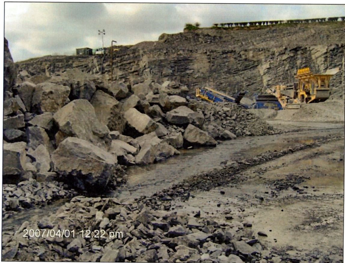
Quarry in operation in 2007 (water pipes in background – facing toward canal bank).
