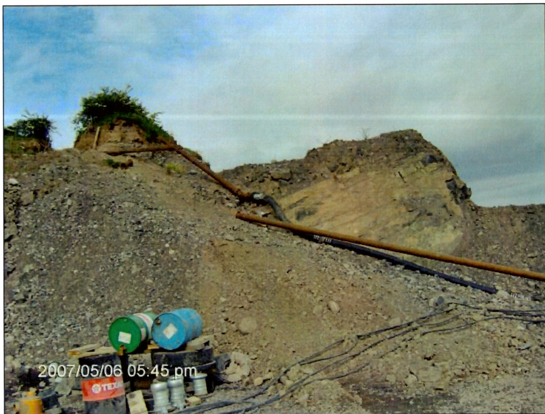
Water pipes and fuel tanks exposed in quarry.
